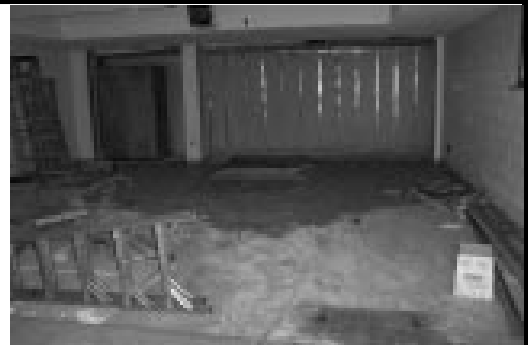
One of our first goals was to install a support system for underneath the new baptismal
